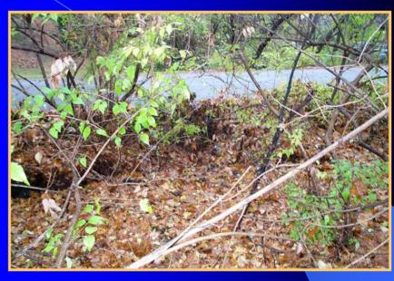
Remove leaves and debris from ditches, culvert pipe openings and storm inlets before drainage is blocked. Periodically removing small amounts of debris is a more manageable process.
