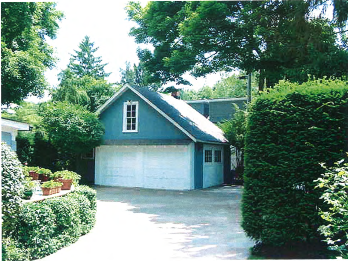
Figure 27. Garage north & west façades. WLS, 2004.
