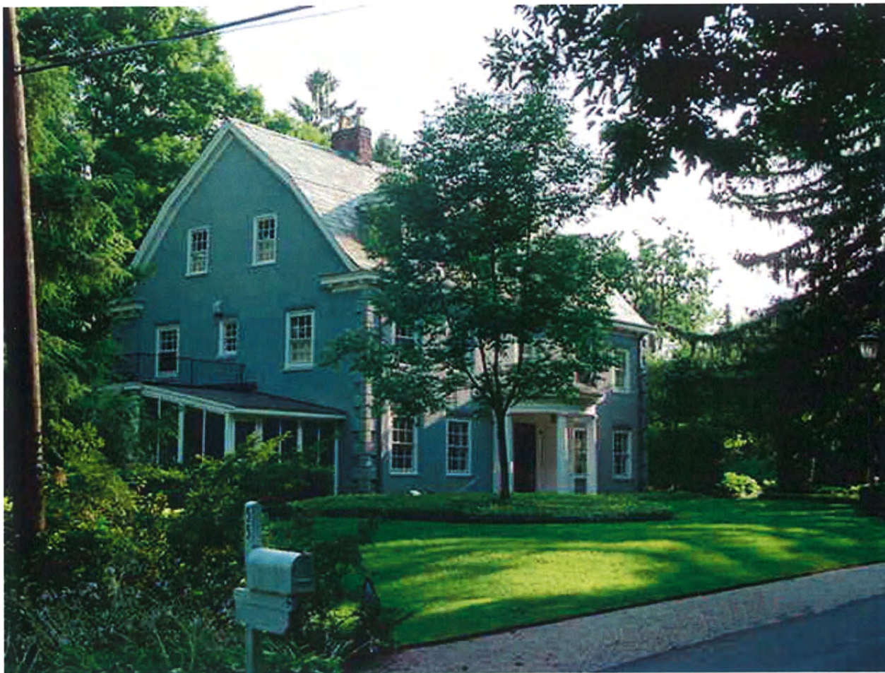
Figure 6. North and east façades. WLS, 2004.
