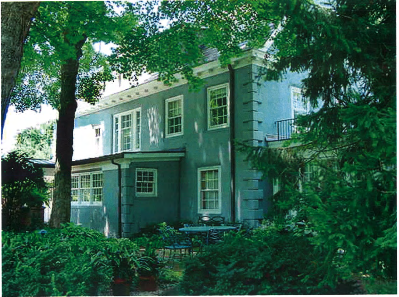
Figure 12. Detail of south façade showing addition. WLS, 2004.
