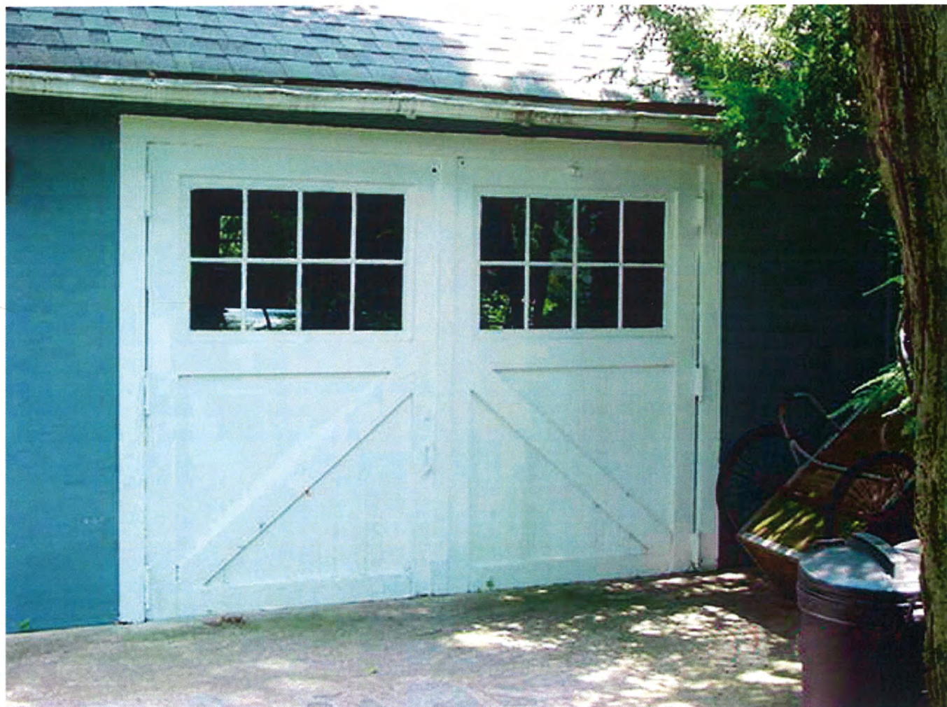
Figure 28. Original 1924 garage doors on west façade. WLS, 2004.
