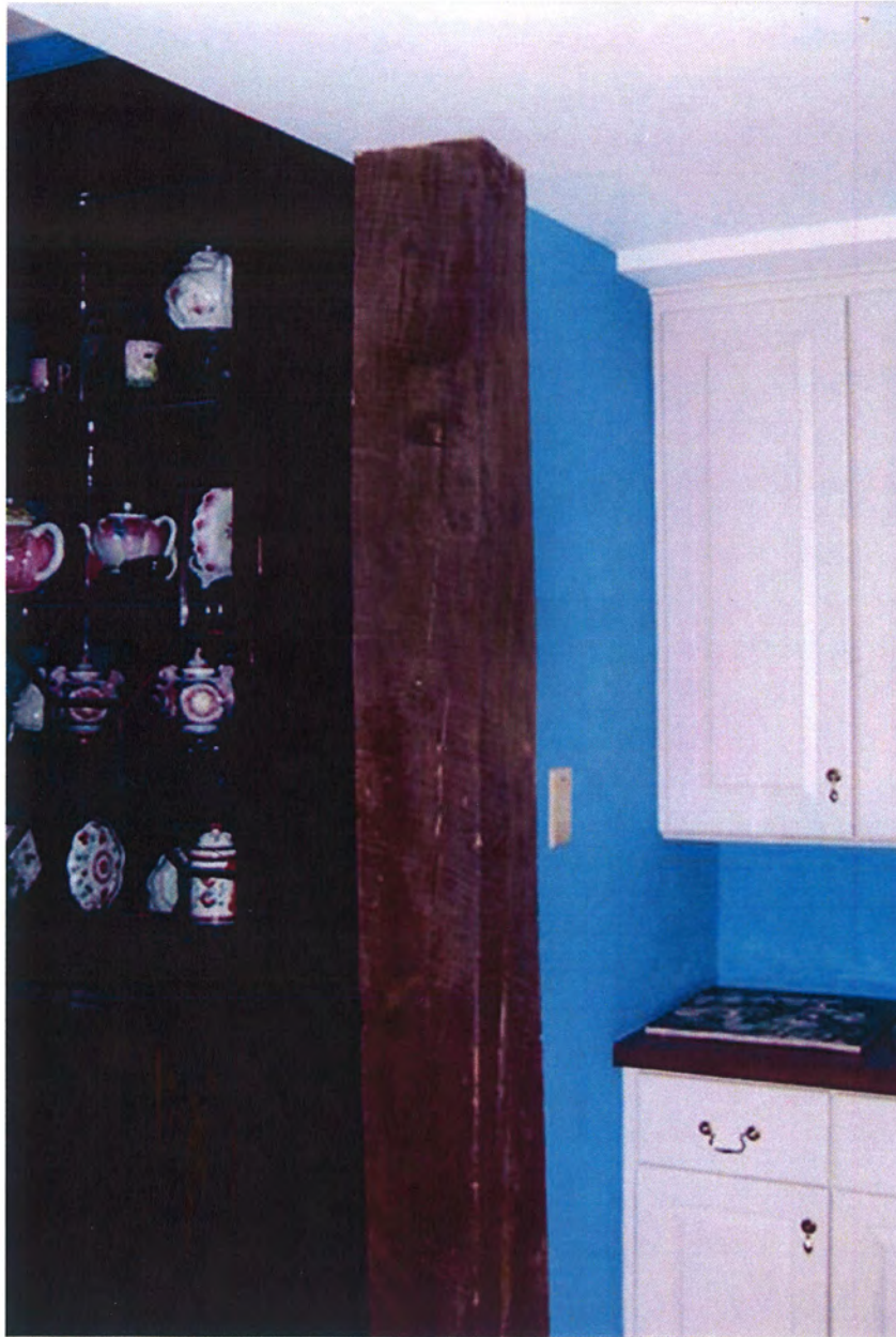
Figure 2. Exposed heavy-timber post on third floor. WLS, 2004.
