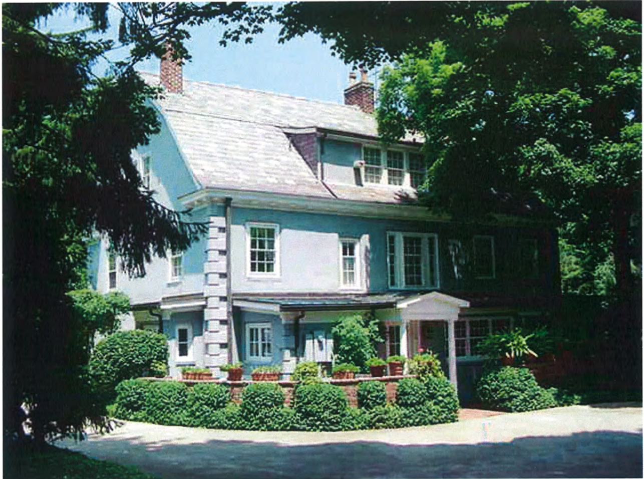
Figure 7. South (rear) façade showing the first floor addition. WLS, 2004.
