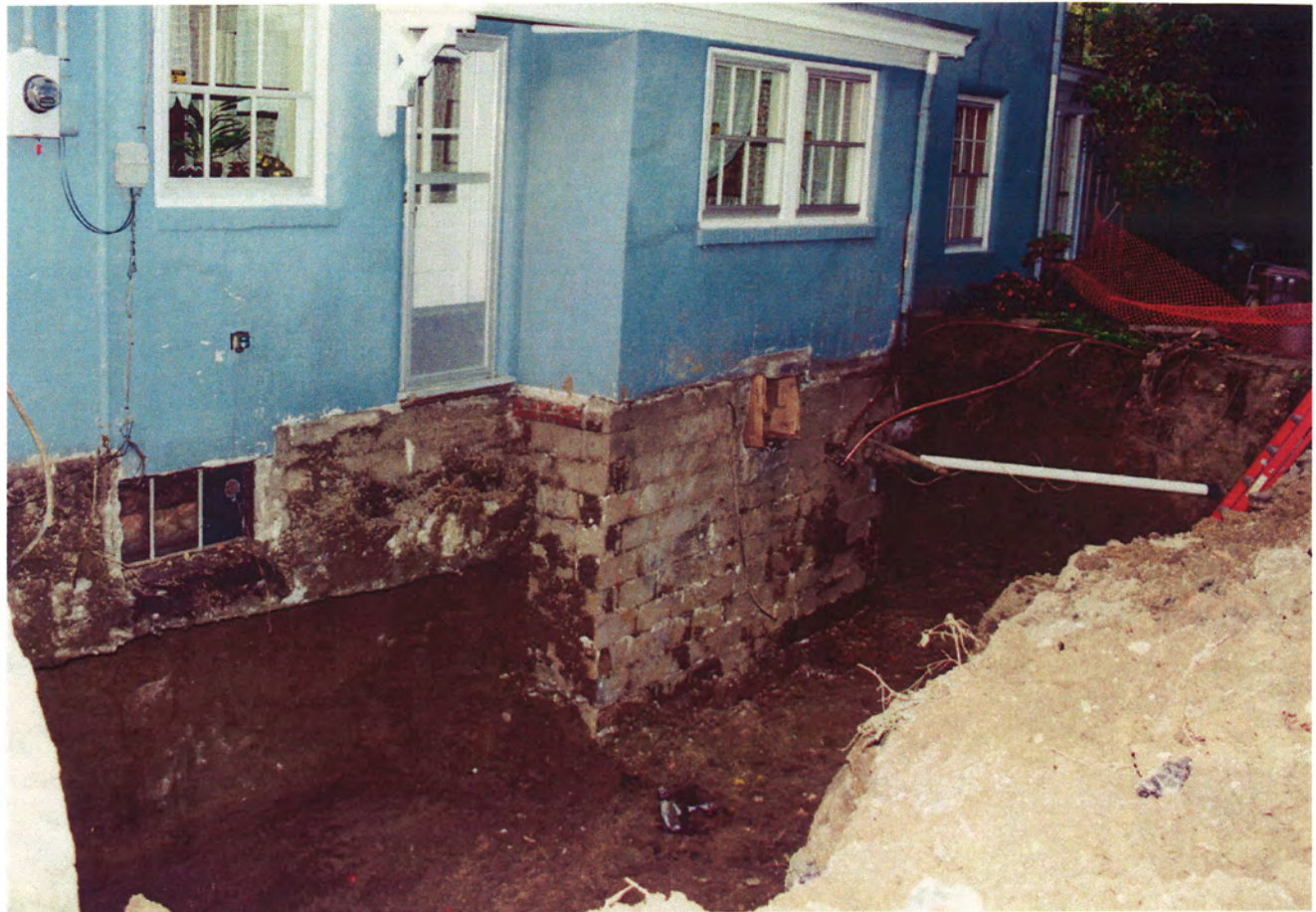
Figure 34. South façade foundation excavation. T. Mueller, 1993.
